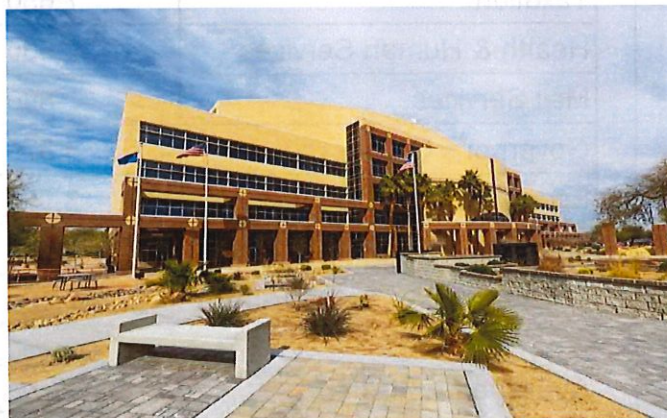
Grant Sawyer Building, Las Vegas
